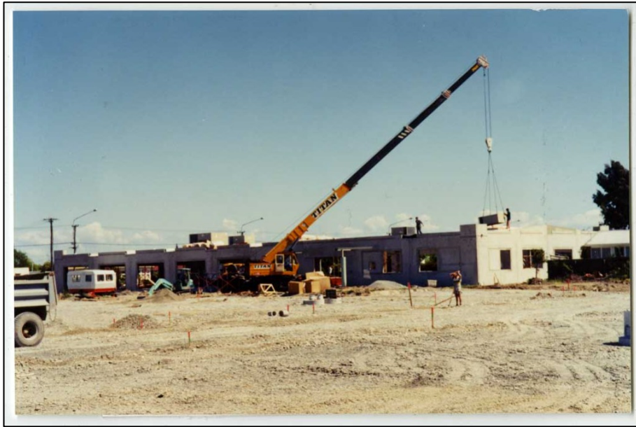
2 nd Shirley Library construction 148
