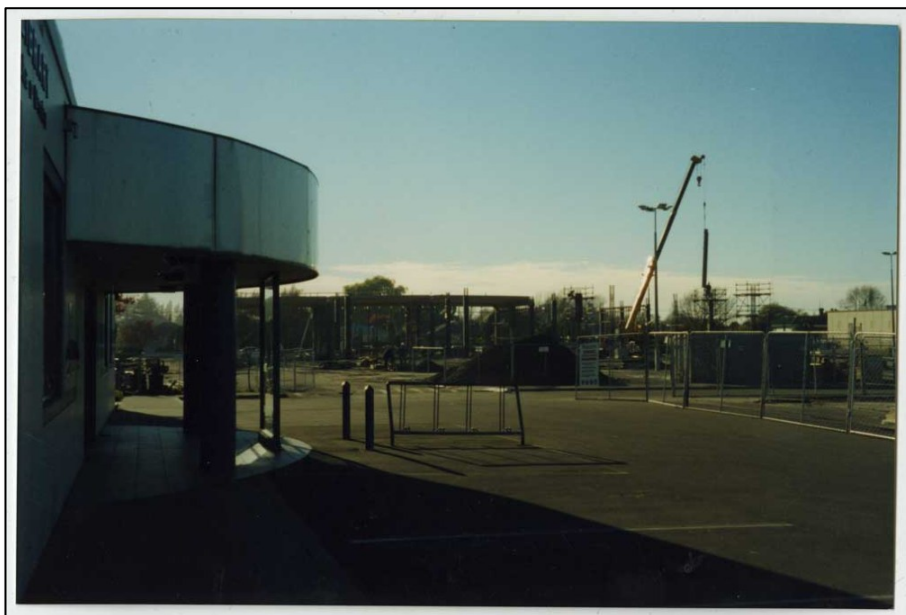
2 nd Shirley Library with The Palms mall construction 151
